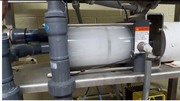
Polyblend® Magnum Mix Chamber with Two Zone Mixing
