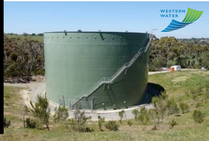
Western Water's Rosslyne Water Filtration Plant Storage Tank
